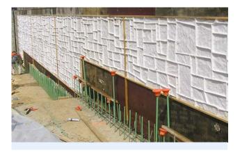
Sika thermoformed plastic formliners are used for texturing tilt- up, cast-in-place or precast architectural concrete. Sheets of formliner attach to the formwork or casting bed prior to placing the concrete. Following placement and normal curing time, the formwork and formliner are stripped, leaving a textured concrete surface.
