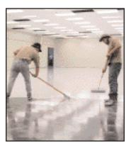
solvent free epoxy was applied as a quartz sand filled, self smoothing floor finish. After 24 hours curing, all building movement joints were prepared and filled with Sikaflex 2C, a two component, polyurethane joint sealant.
