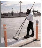
An abrasion resistant, polyurethane, Sikafloor 455 was applied and broadcasted with quartz sand to act as a slip resistant finish. After 24 hours all unbound sand was removed and a further coat of Sikafloor 455 was applied to encapsulate and seal the sand into the surface.
