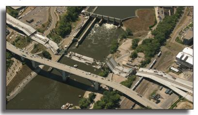
deck truss construction while all but two of the eleven approach spans were steel multi-girder construction, the two exceptions being concrete slab construction. The bridge ranked as Minnesota's fifth busiest and carried more than 140,000 vehicles a day. It was estimated that the loss of the bridge resulted in \$400,000 per day in lost revenue, increased commuter expenses and stress on surrounding roads.
