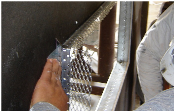
Typical CI Weep Track at Opening
