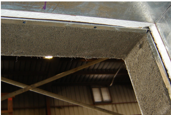
Typical Opening/Return after Stucco Application
