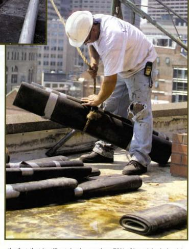
the fact that it still retained more than 70% of its original plasticizer content, it was decided that with the scope of work related to the masonry and the magnitude of flashing work to be completed, it would be prudent to replace the roof as well. This would establish a continuum of the building envelope to assure the desired level of performance.
