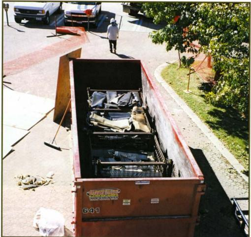
Figure 9 - Old membrane packaged in dumpster for shipment.
