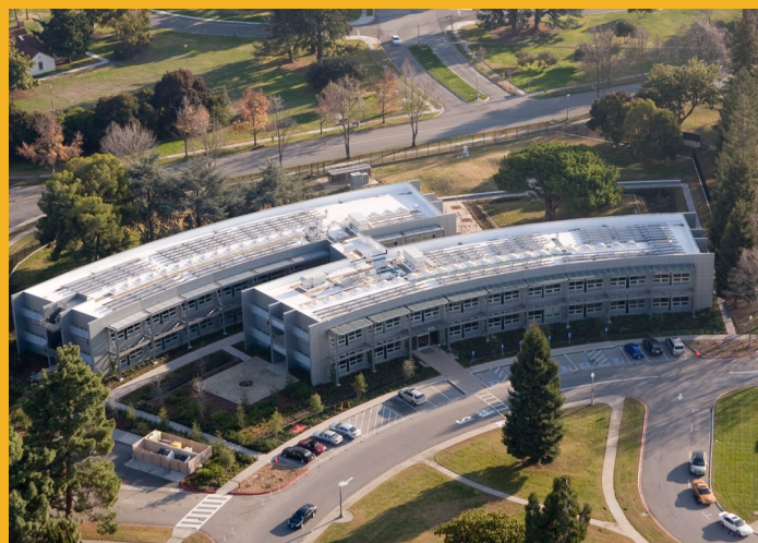
NASA's Sustainability Base in Moffett Field, California, is considered the federal government's "greenest" building and features a Sika Sarnafil EnergySmart Roof®.
