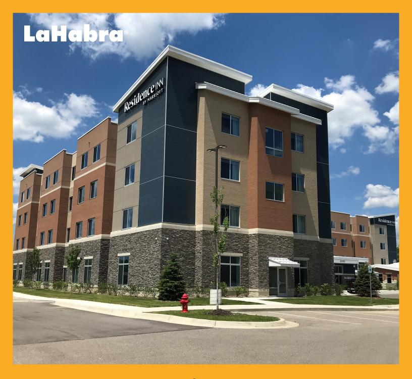
Cement Board System with Adhered Veneer
