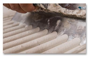
**Latex Portland Cement Grout** - combines Portland cement grout with latex additives for increased performance.
