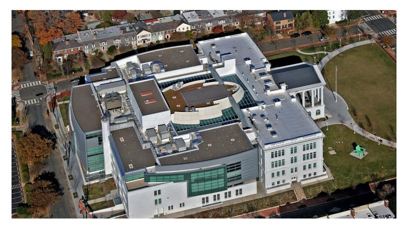
checks at each point to ensure that the area around each obstruction achieved drainage. HRGM also had to restore and reconfigure the half-round, built-in gutter at the front of the building, without making visible changes to the facade. This was accomplished by end-damming select sections of the rebuilt gutter, lining the full gutter with Sarnafil 80 mil membrane, and resloping the adjacent roof sections using carefully aligned crickets and insulation fill.
