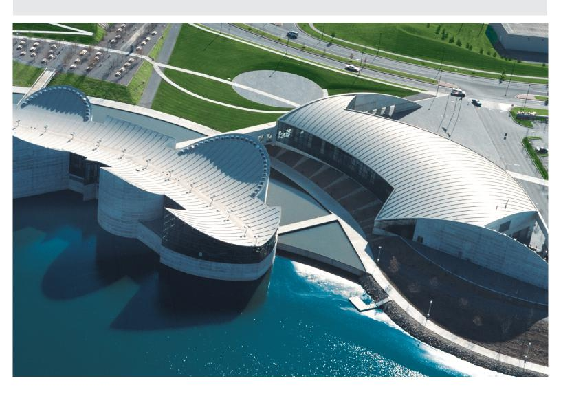
"THE POWERFUL GEOMETRIES OF THE ISLAND AND LAND WINGS OF EXPLORATION PLACE REQUIRED A ROOFING SYSTEM THAT WOULD LEND ITSELF TO THE POSITIVE AND NEGATIVE TOROIDAL FORMS OF THE ROOFS."
