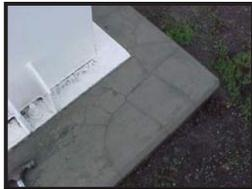
Exposed shoulders in portland cement grouts can develop cracks. When shoulder cracks occur
