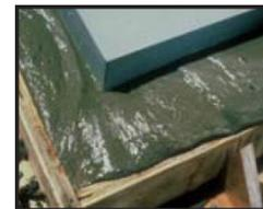
Shoulders do not serve a structural function for precision grout; they are essentially a construction requirement.
