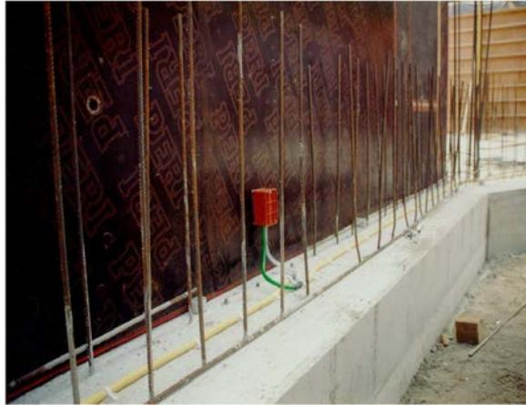
Figure 2: vent ends entering junction box
