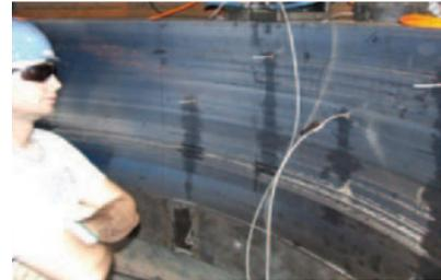
3. Inject SikaFlow®-647 Grout through the fittings/ports into the void until any water or oil has been flushed out and the grout is discharged from the crack.
