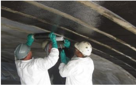
EXTERNALLY BONDED FRP OR STEEL
