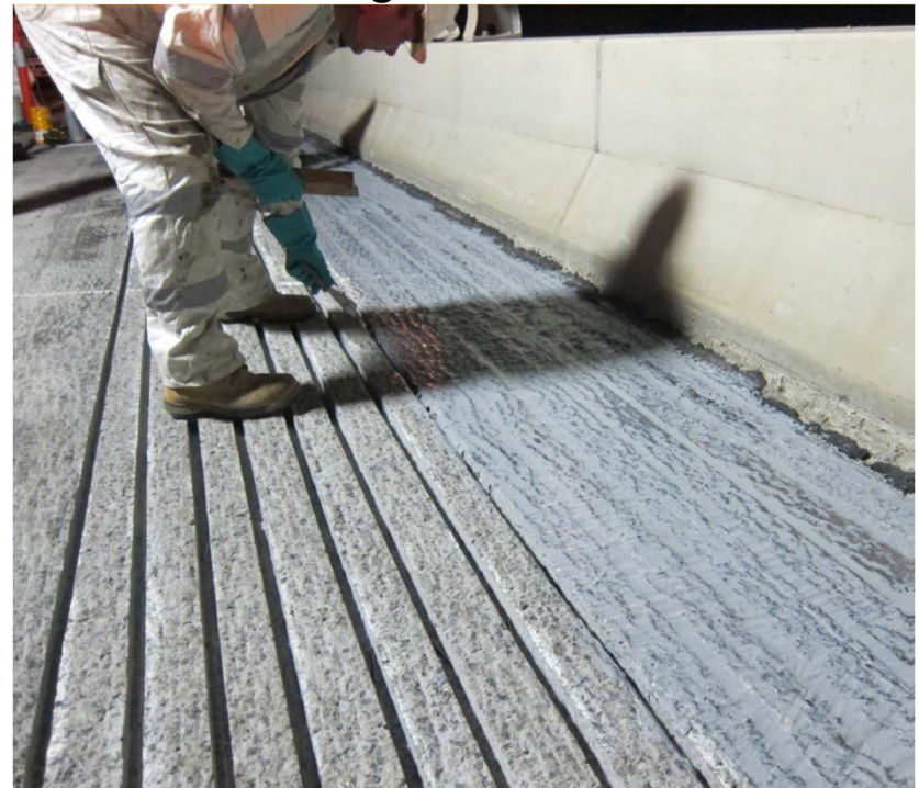
Place rods in the groove
