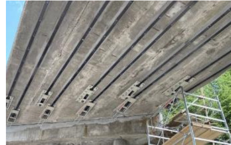
EXTERNAL POST- TENSIONING
