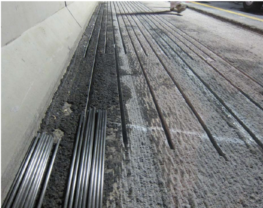
Cut and clean grooves
