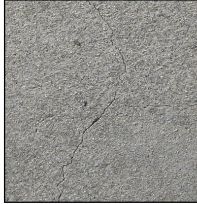
Hairline cracks on a stucco wall
