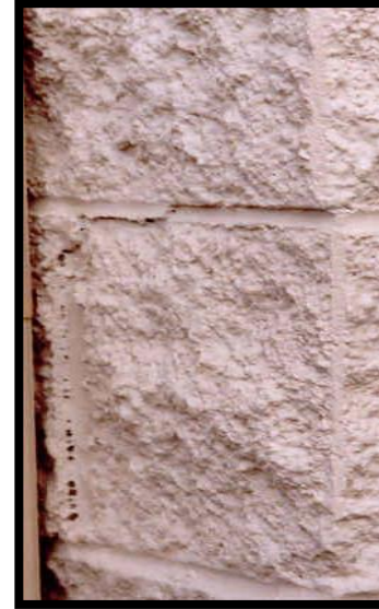
Structural Settlement Shrinkage
