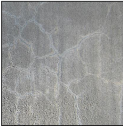
Surface cracks on a precast panel
