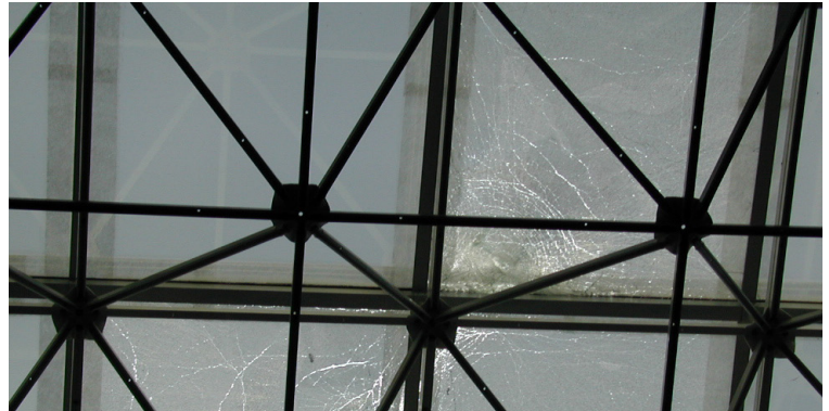
Skylight was protected with Sikalastic® Clearglaze. After a hurricane event, the skylights shattered but remained in place
