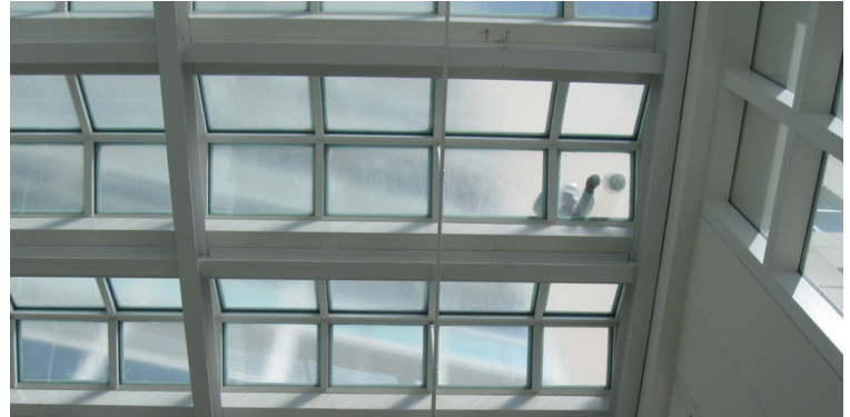
Appearance of Sikalastic® Clearglaze applied to existing skylights
