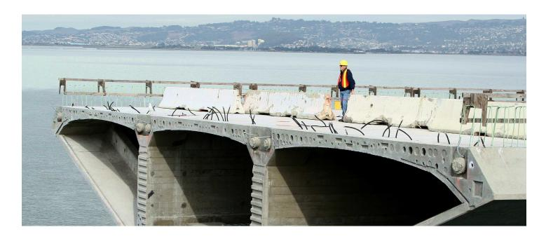
Build and protect your civil and commercial projects year round with Sikagard and Sikadur materials. Sika's high performance epoxy Segmental Bridge Adhesives (SBA) are high-modulus, high-strength and low creep even at low temperatures. Sikagard protects the surface from chloride intrusion and corrosion from de-icing salts used heavily in winter months as well as increasing longevity of marine structures.
