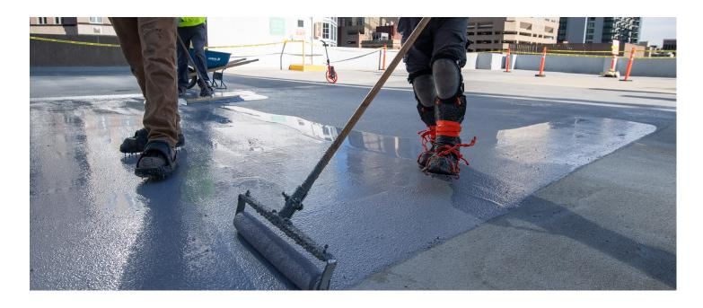
Sika provides comprehensive solutions to waterproofing problems with maximum protection. Sika's wide range of traffic coatings are designed to make concrete and masonry impermeable to water, while offering flexibility to handle all of your park deck waterproofing needs.
