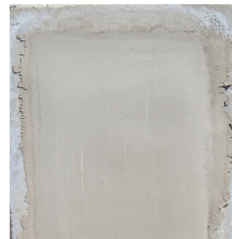
Finish with trowel, float, or sponge, depending on desired surface texture.
