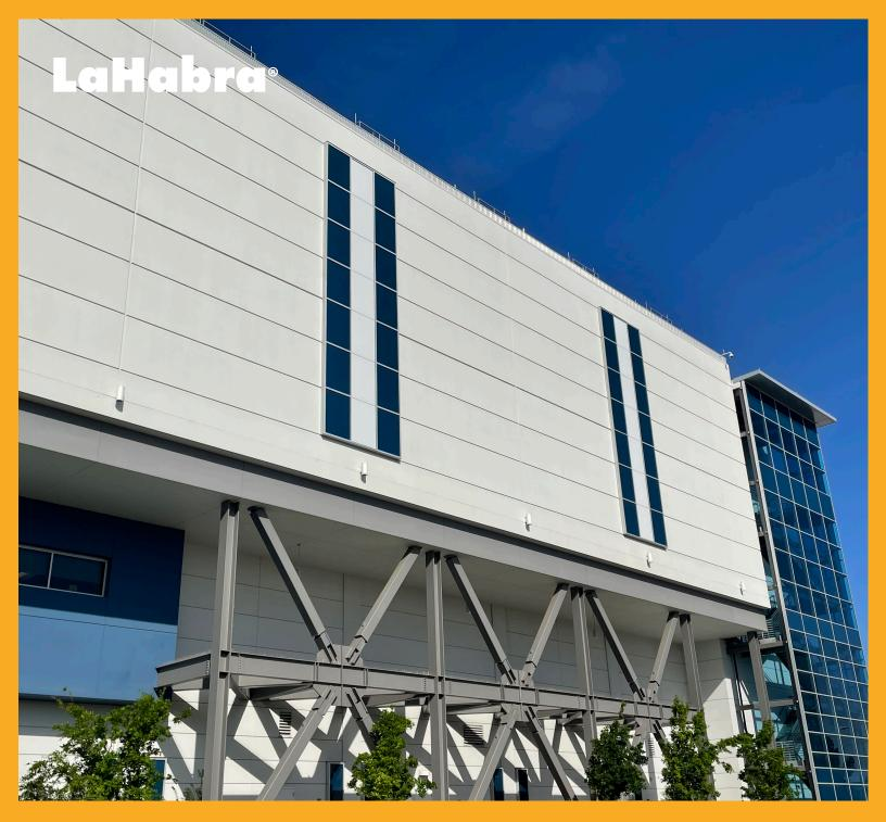
Premium Cement Plaster Stucco with a Finestop Fluid Applied Air/Water-Resistive Barrier
