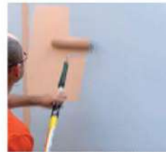
Fig. 6. Coating application with proper overlap
