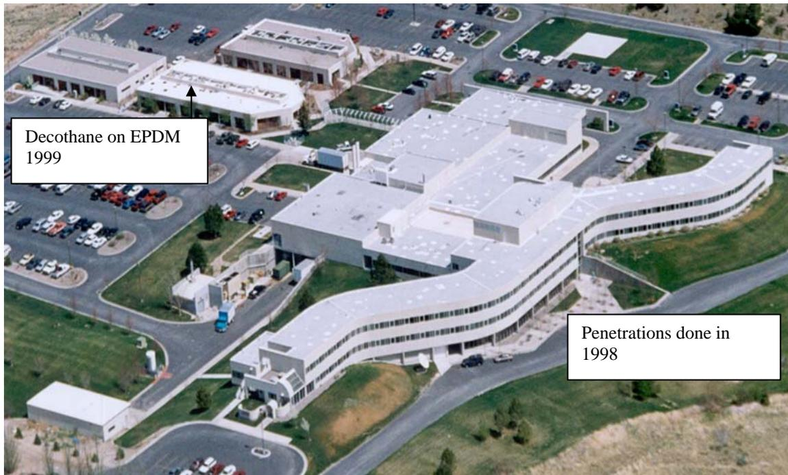
**Picture taken Spring of 2000. Note Medical Office Building EPDM Roof and Decothane on main hospital roof.**
