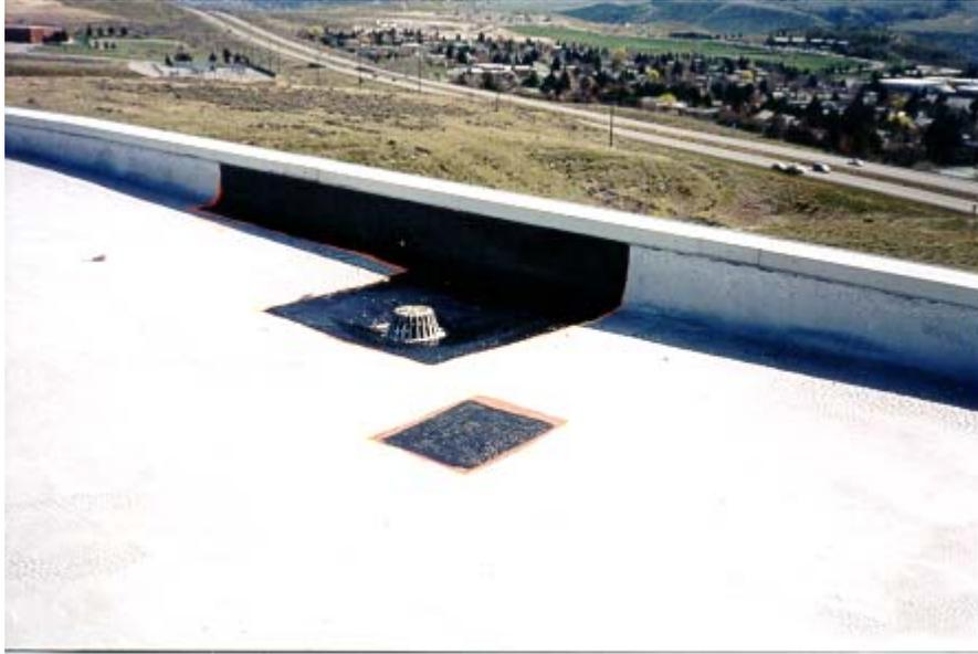
PHOTOGRAPH NO. 3 – OVERALL VIEW OF DRAIN AND PARAPET REPAIR
