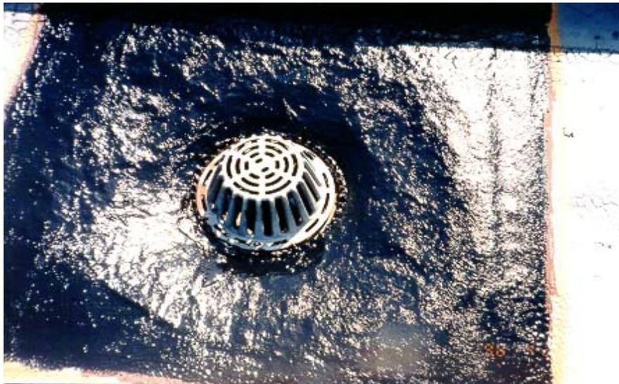
PHOTOGRAPH NO. 4 – CLOSE-UP VIEW OF DRAIN REPAIR
