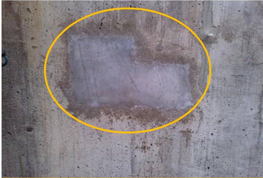
Concrete Spall Repair
