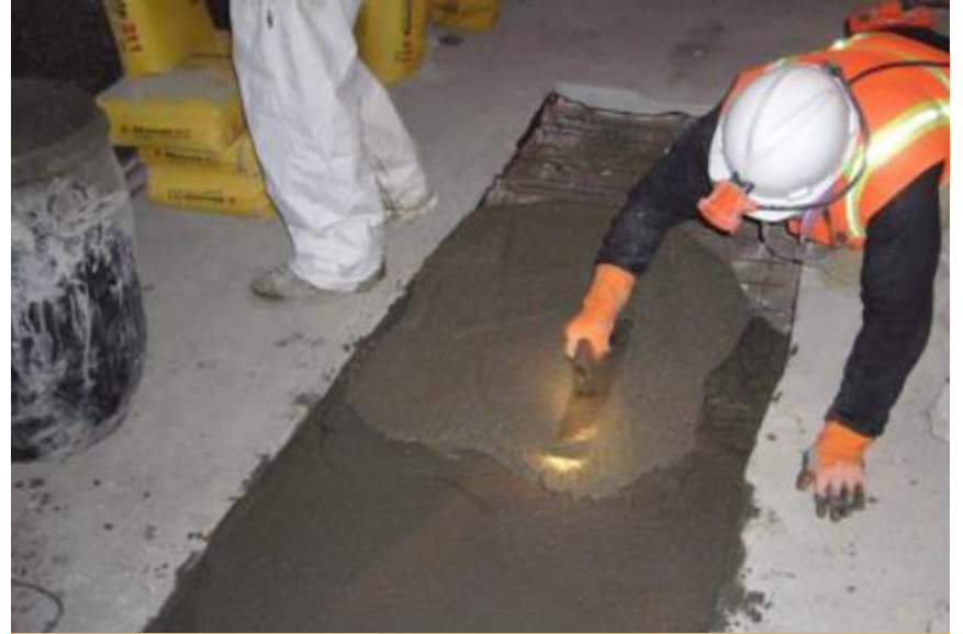
Repair Spalls
