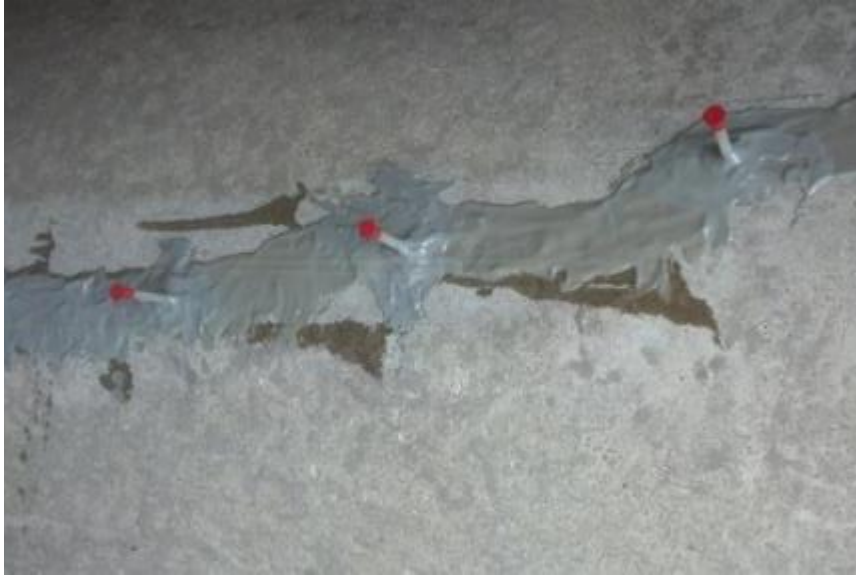
Inject Cracks with Epoxy
