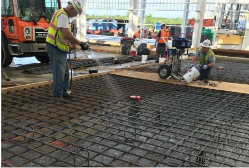
Clean Rust and Treat Exposed Rebar
