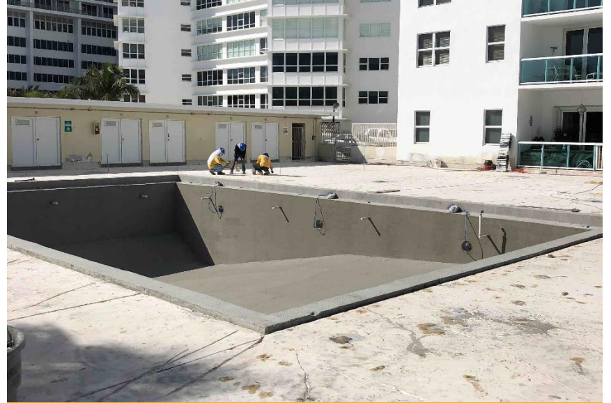
Waterproofing of Pool Basin
