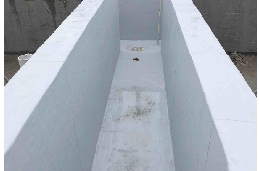
Water Test on Planters After Waterproofing Membrane Application
