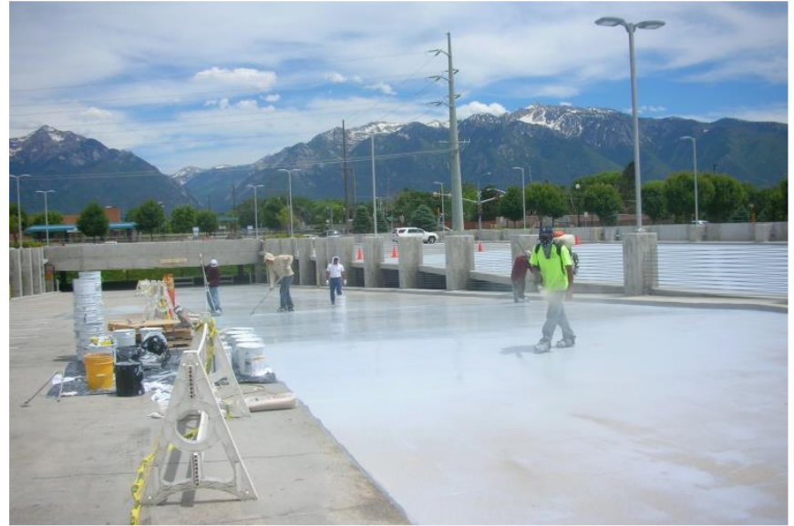
Replace Deck Coating
