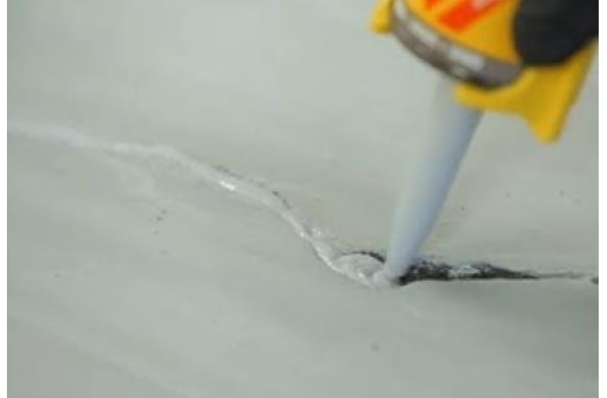
Rout and Seal Surface Cracks
