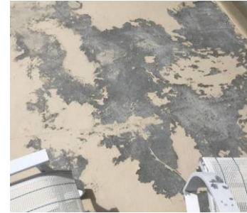
Waterproofing Failure
