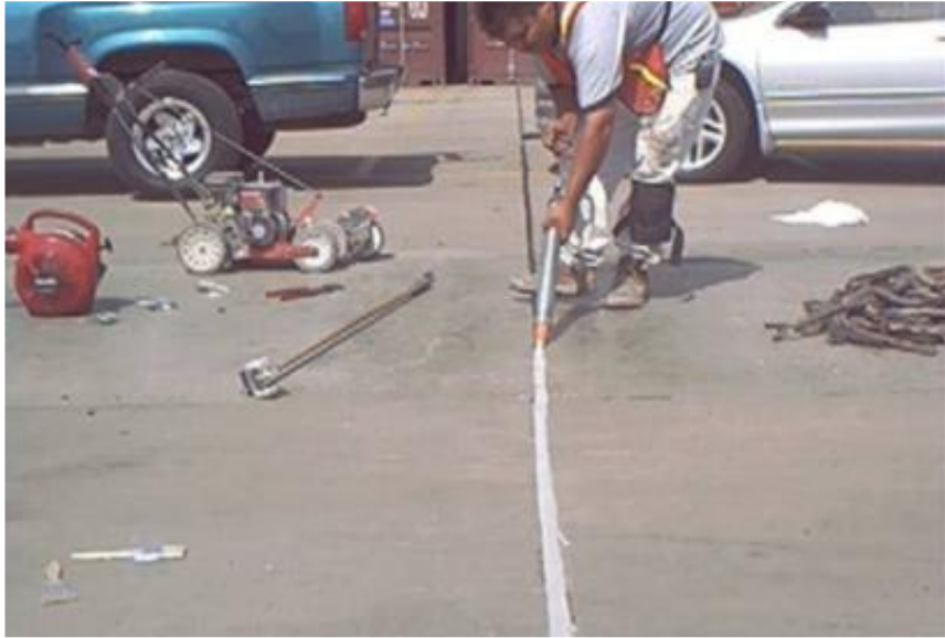
Replace Deteriorated Joint Material
