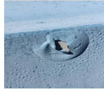
Waterproofing Failure
