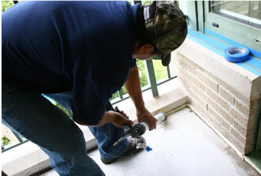
Joint Sealant Replacement
