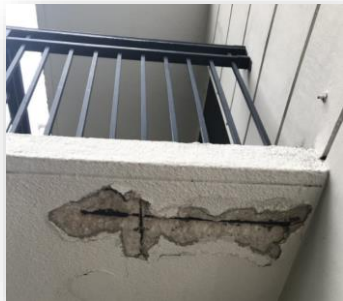
Spalling Concrete
