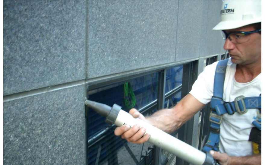
Ensure Sealant is Properly Installed
