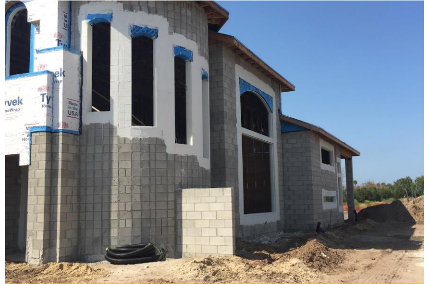
Window Waterproofing Flashing
