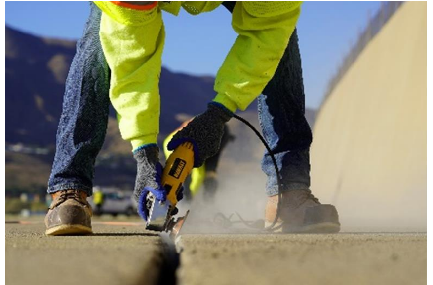
Preparing Joints for Sealing
