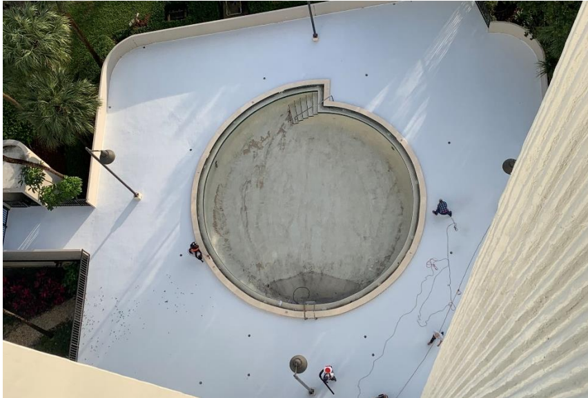
Application of Waterproofing Membrane on Pool Deck
