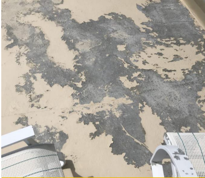
Waterproofing Failure
