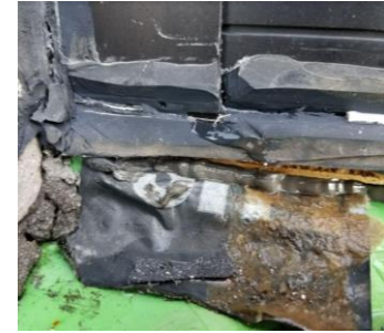
Waterproofing Failure
