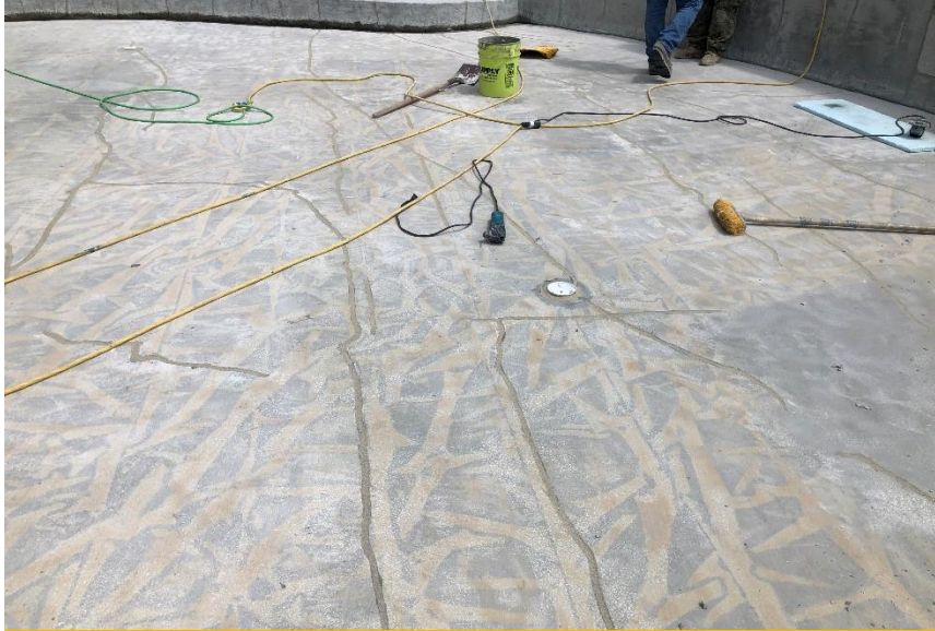
Crack Sealing Inside Pool Basin
