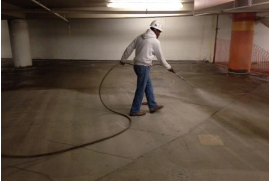
Surface Applied Corrosion Inhibitor
