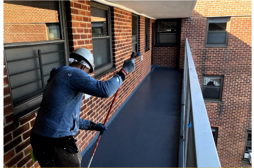
Waterproofing Replacement
