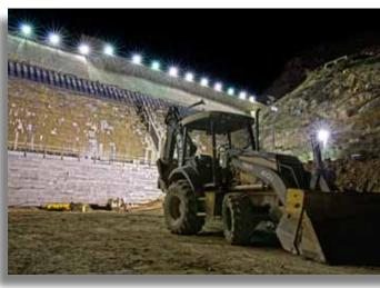
Layers of roller-compacted concrete 24 inches thick completely cover the downstream side, producing a stairstepped surface. The new concrete is nearly equal in volume to the original dam.
