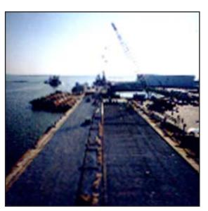
The purpose of the project at the Port of Wilmington (DE) was the extension of one of the ports piers. Since the chlorides in the seawater can cause, even at an early stage, corrosion of the reinforcement bars in the concrete, the contact with seawater reduces the service life of concrete structures significantly.
