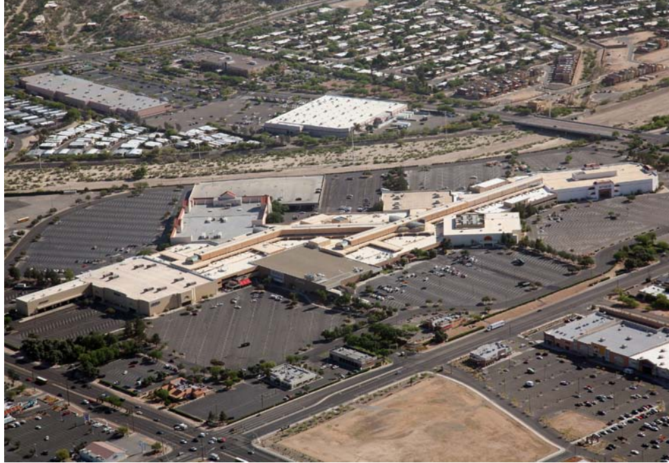
Pictured is the Tucson Mall. In 2007, Clark’s Quality Roofing was awarded the Sika Sarnafil Century Award — signifying 100 Sika Sarnafil installations within a calendar year — for the fourth consecutive year.
