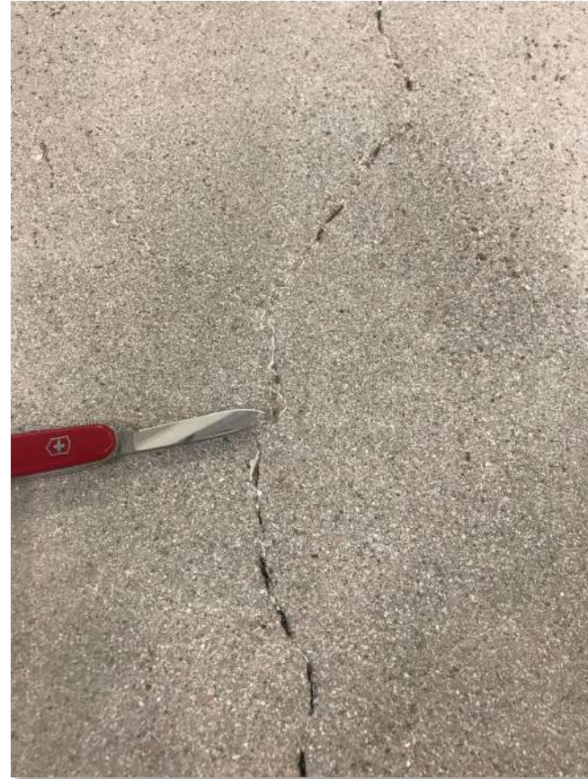
After shot/sand blasting
