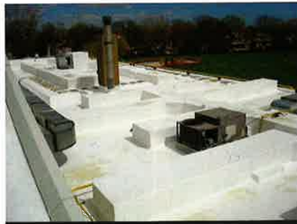
Studies estimate that modest increases in urban roof reflectivity could generate billions of dollars of economic prosperity for cities. Pictured here is the roof on the Cricket Club in Toronto.
