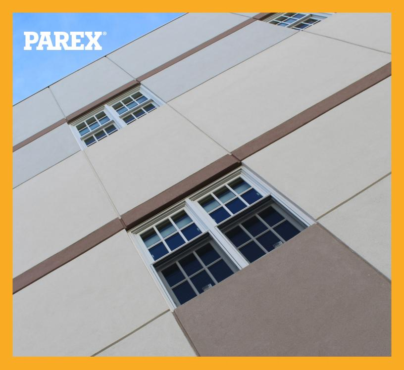
Weather-resistant cladding consisting of a mesh-reinforced base coat and acrylic finish over a structurally insulated panel.
