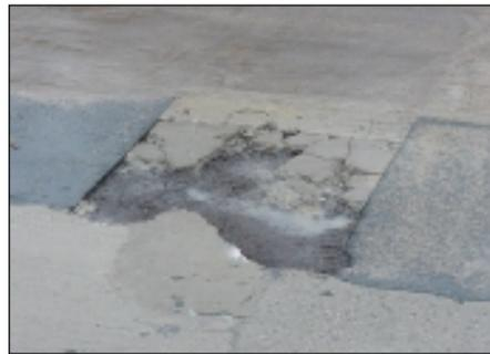
Spalling of concrete on the bridge deck led to an investigative analysis. The analysis indicated that the quality of the concrete cover was poor and in many areas insufficient in depth. The bridge is also exposed to an aggressive environment. All of these factors contributed to accelerating corrosion of the reinforcing steel which led to spalling of concrete in various areas throughout the deck.
