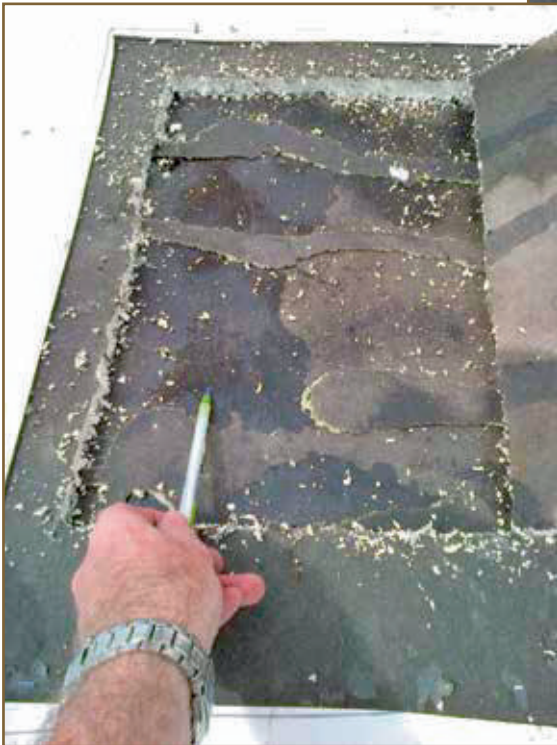
Photo 10 – Moisture between the layers of iso.
