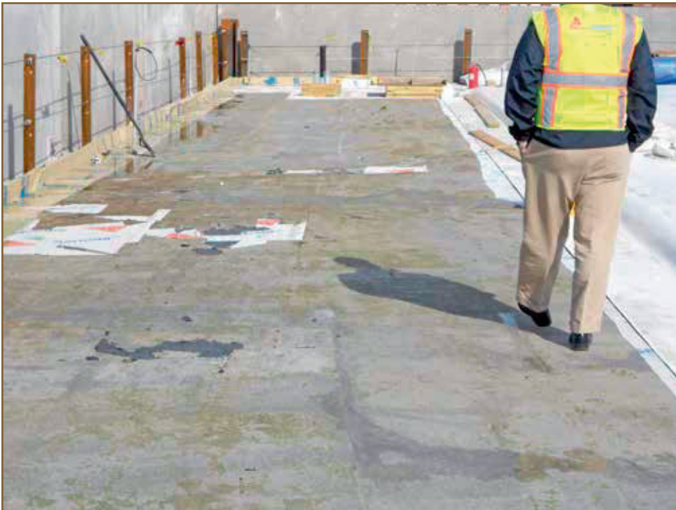
Photo 6 – Roofing removed from the perimeter.
