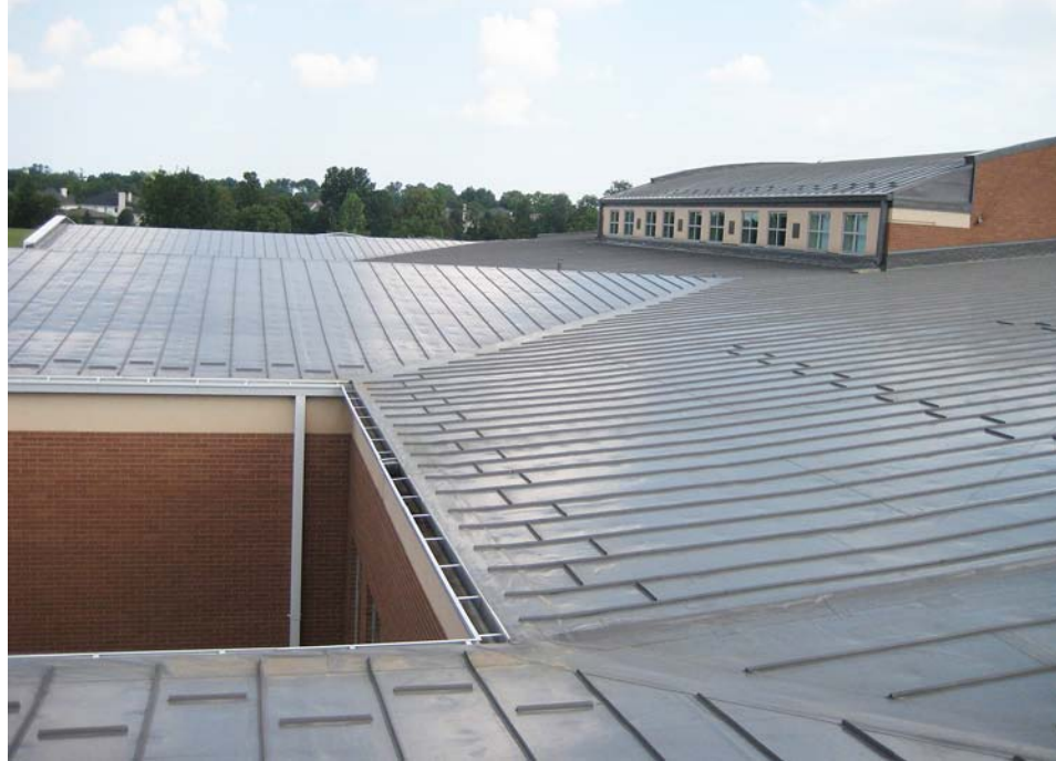
The flexibility inherent in the Décor Roof System made the job of Midland Engineering, the roofing contractor, easier when faced with the many flashing details, elevation changes, valleys and roof configurations at the Smoky Row School.
