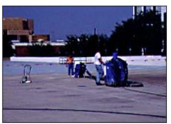
This post-tensioned parking structure measures over 125,000 square feet on only one level. Cracks and failed joints caused severe leaking into the covered parking below. A number of areas had ponding water that made the leaking worse. This leaking water caused problems in the occupied space below. With a number of high-profile clients in the building, the owner determined that an aesthetic waterproofing system was needed to protect the concrete and the tenant's cars.
