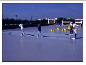
to slope the concrete surface to the drains. After leveling was complete, all cracks were routed and sealed using Sikaflex 2c, Sika's two-component polyurethane joint sealant.
