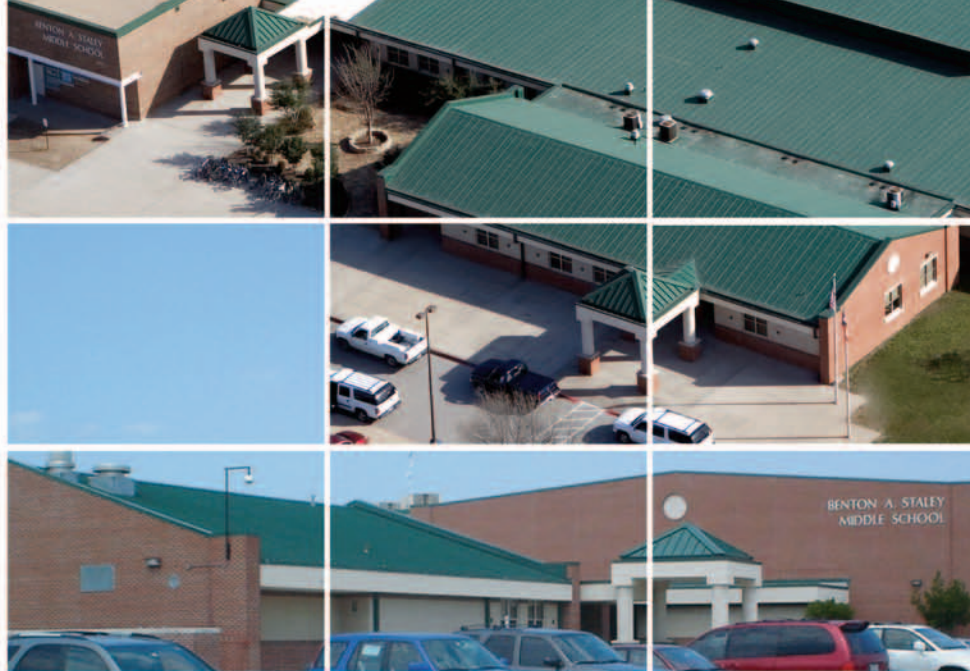
Sarnafil Décor Roof System on the Staley Middle School in Frisco, TX
