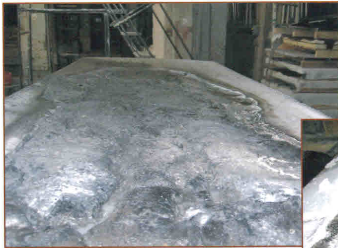
Photo 8 - TPO over isocyanurate.
