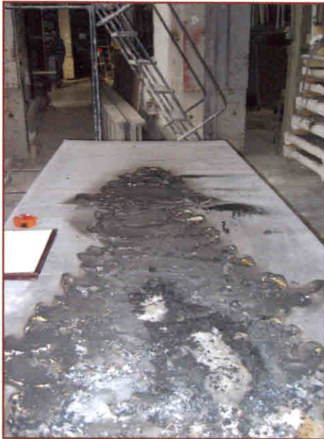
Photo 4 – FR-rated EPDM over listed gypsum board.
