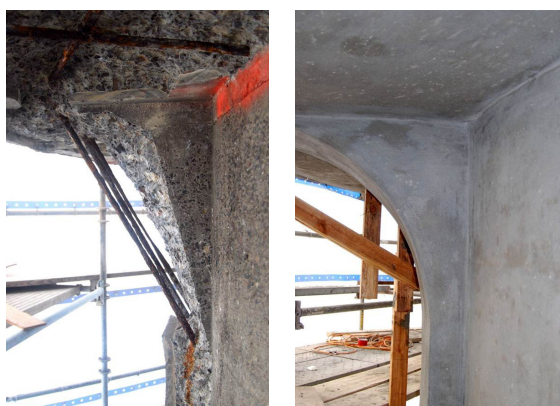
A cornice support before and after protective coating applied
