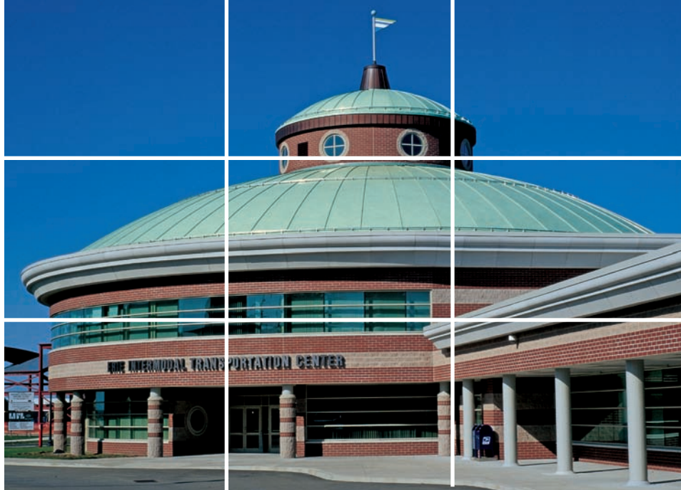
Roofing Contractor A.W. Farrell & Son began work on the Erie Intermodal in a November, and the bitter winter months typical to the Erie area that followed made for arduous work conditions.
