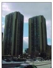
River. This case study focuses on two 38 story apartment buildings which were constructed between 1970 and 1972. Inspections conducted in 1997 identified numerous areas of spalls due to corrosion of the steel reinforcement. More recently, sealant joints at the sliding glass doors, ac units and windows were failing and allowing water to leak into the apartments.
