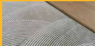
FLOOR COVERING INSTALLATION
