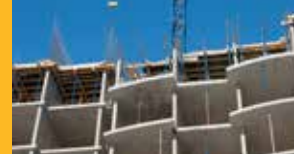
CAST-IN-PLACE & PRECAST CONCRETE
