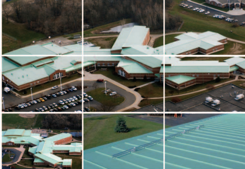
Mount Vernon Middle School, Mount Vernon, OH - Sika Sarnafil's 2006 Roofing Project of the Year
