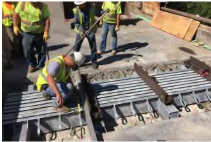
JOINT SEAL ASSEMBLY
