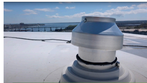
Wind Vent Valve photo taken above the Holiday Inn Riverview in Charleston, SC
