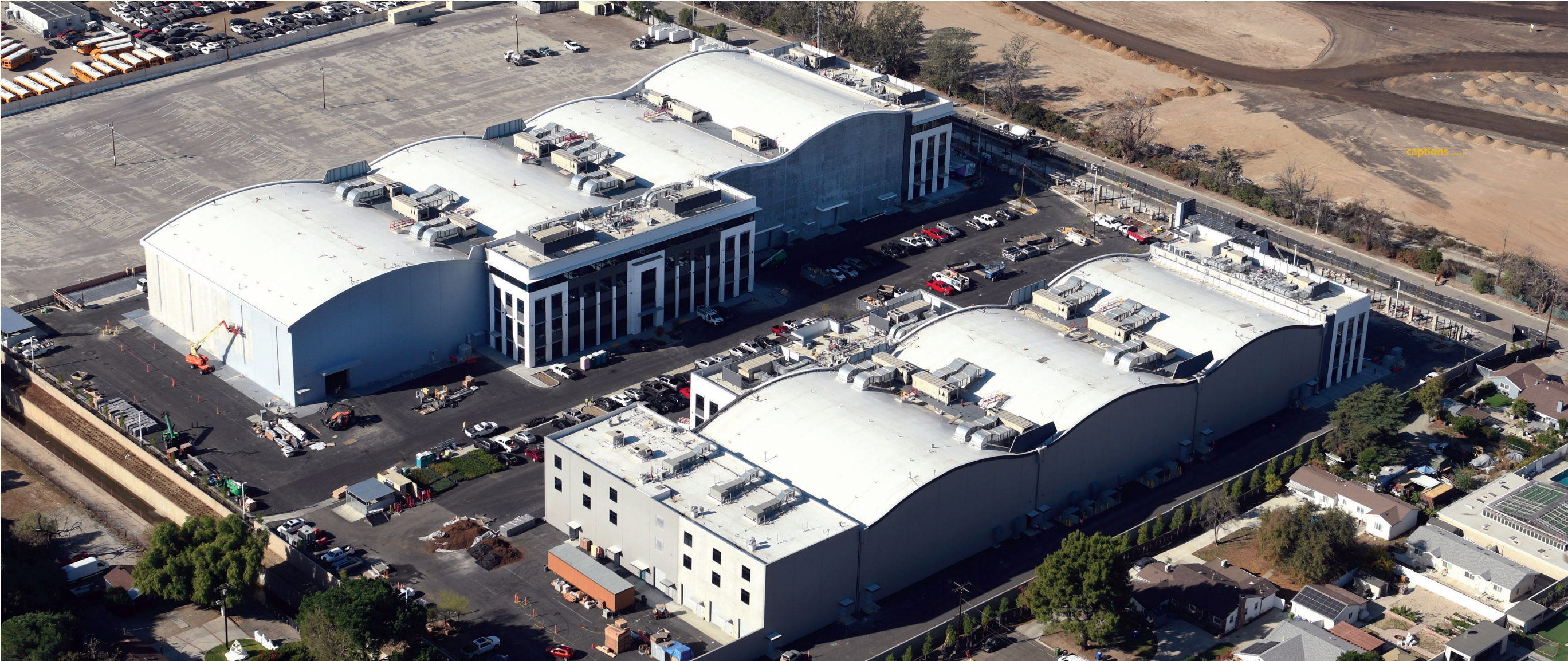
For the roofing membrane at Sunset Glenoaks Studios in California (above), the project team used Sarnafil G 410 60-mil, Energy Smart Reflective Gray. It was fully adhered using the low-VOC water-based Sarnacol 2121 adhesive. At right, Sika's first post-consumer recycling project, the Marriott Long Wharf in Boston, was completed in 2005.
