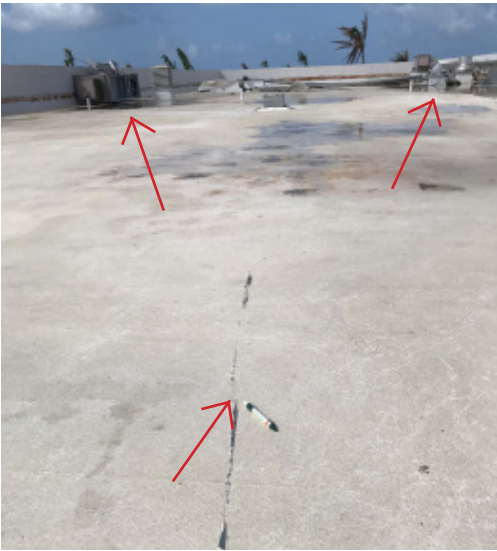
Mechanical equipment that became airborne on the CEP building during the hurricane caused skid marks in the Sikalastic membrane
