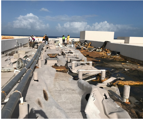
Torn off loose laid membrane system
