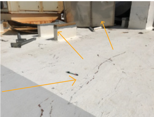
Skid Marks in Sikalastic membrane from airborne debris during hurricane
