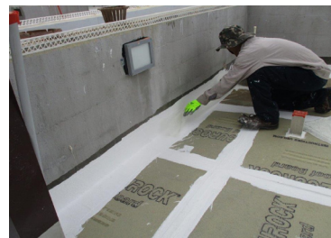
Insulation/Cover Board Installation
