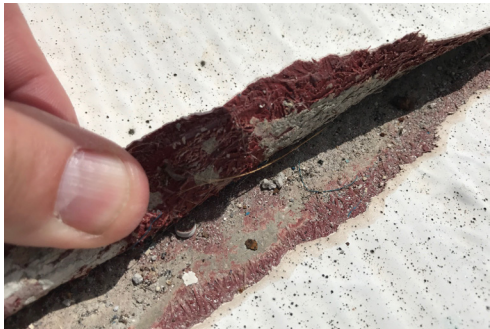
Bonded membrane does not allow water to migrate laterally
