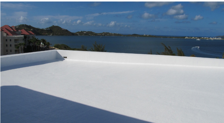
Sikalastic® membrane on the medical building roof at the American University of the Caribbean in St. Martin
