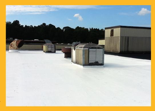
Werner General Contracting then power-washed the roof, and reinforced and repaired areas where needed.
