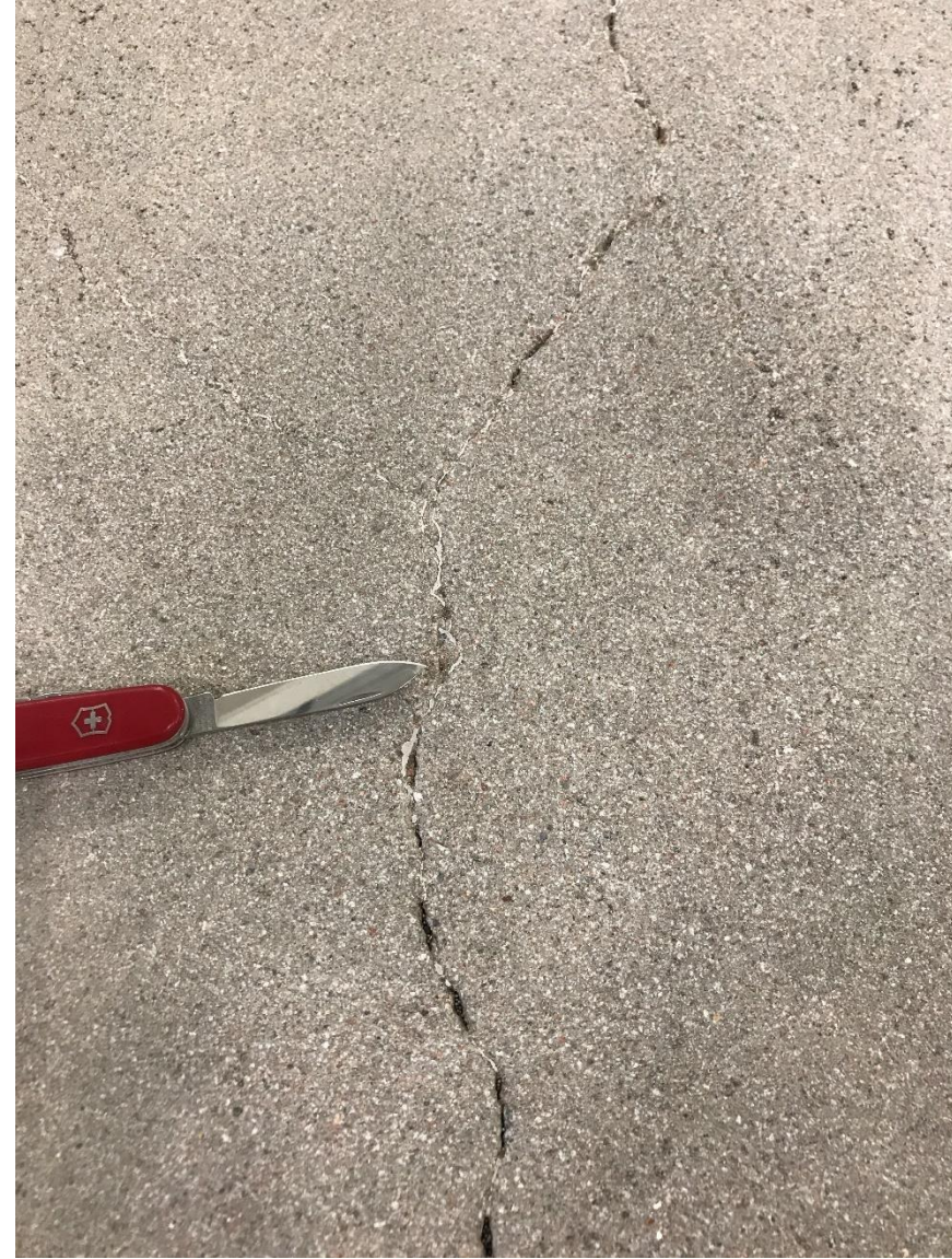
After shot/sand blasting
