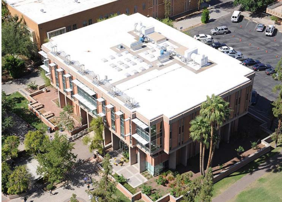
Wind turbines line the front edge of the GIOS roof and solar panels are planned at a later date. The EnergySmart Roof system installed by Progressive Roofing is energy-efficient, will last for decades and can be recycled at the end of its normal lifespan.
