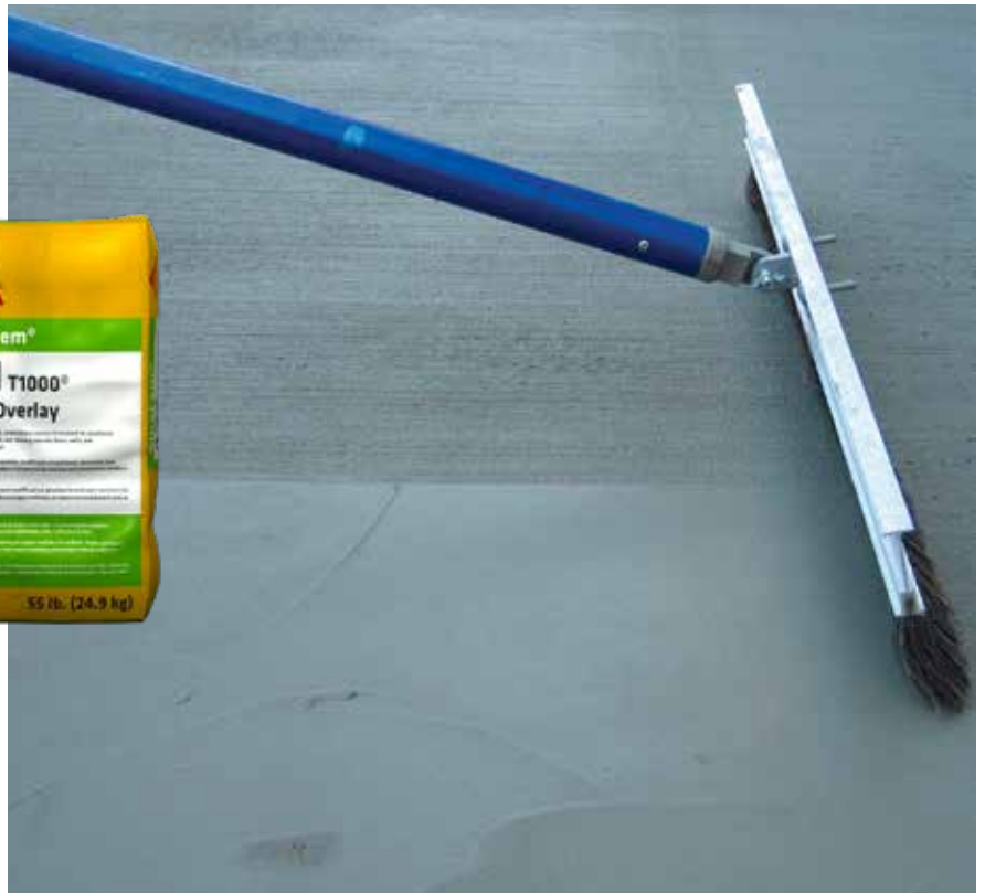
SikaCem®-171 T1000® Fine Overlay Repair Application
