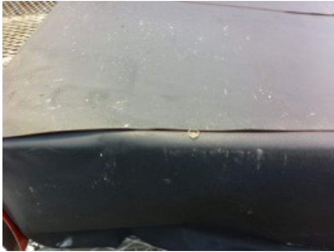
FIGURE 3. OUTER MEMBRANE SURFACE OF TYPICAL SARNAFIL G 476 MEMBRANE AT HARVEST.
