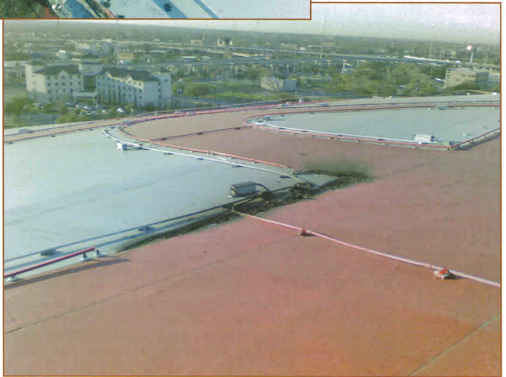
Photo 11 – Overview of roof-mounted lighting system. Fire damage on left side, Toyota Center, Houston, TX.
