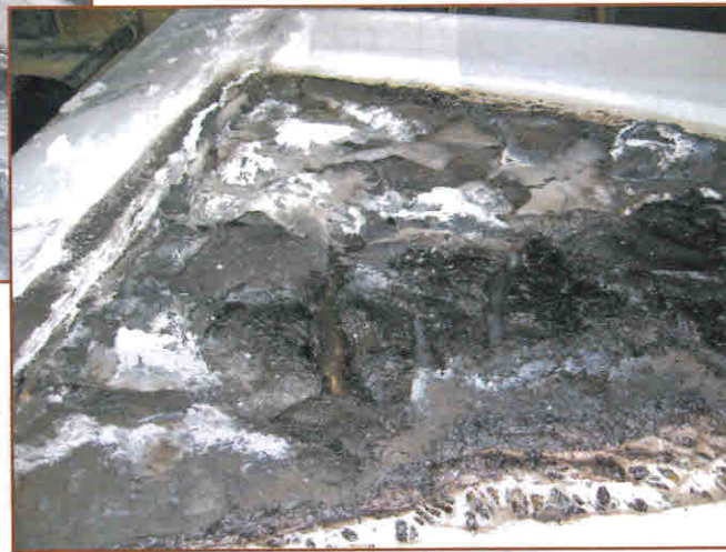
Photo 9 - PVC over isocyanurate, side view.
